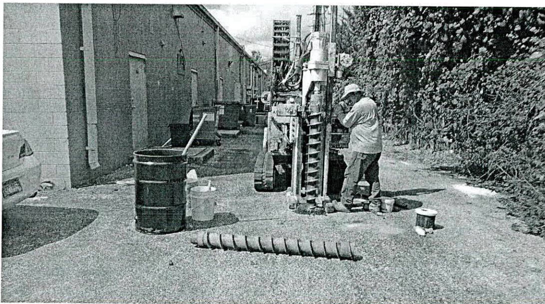
PROJECT: Illinois Ayers Oil Company-Springfield PHOTOGRAPH #6 DATE: 8/30/23 VIEW: West DESCRIPTION: Drilling Monitoring Well PMW-27.
